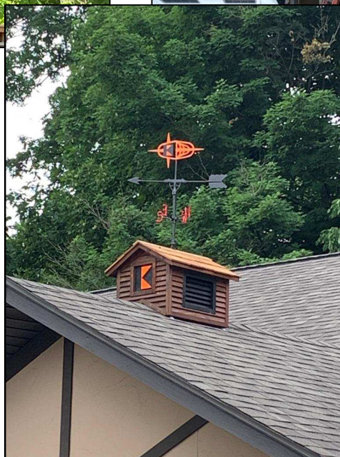
Center, the finished product – the new cupola and Kolping weather vane.
